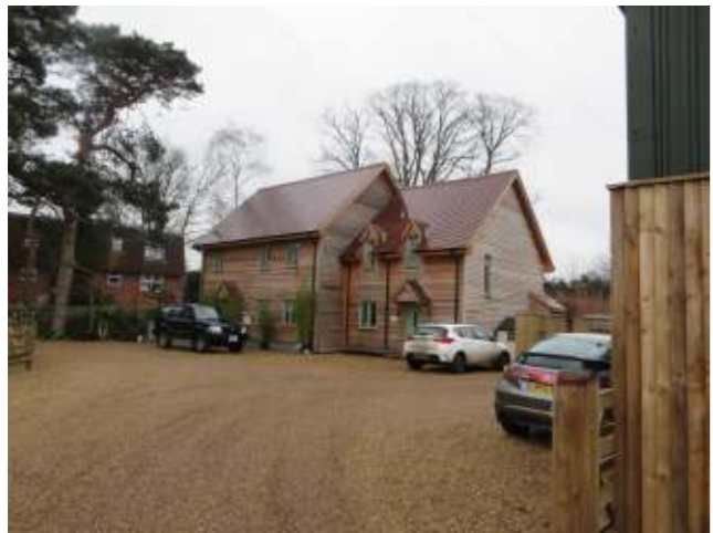
Existing development at the end of Meadow Drive.
