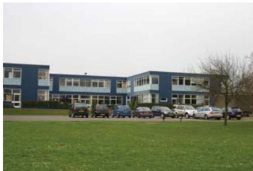
Existing school buildings
