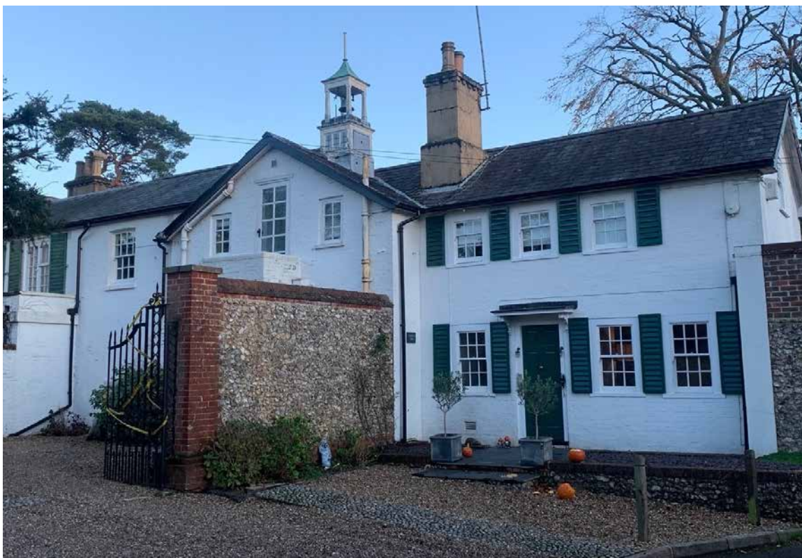
Figure 11: Little Maddison House, formally part of Church Lane House
