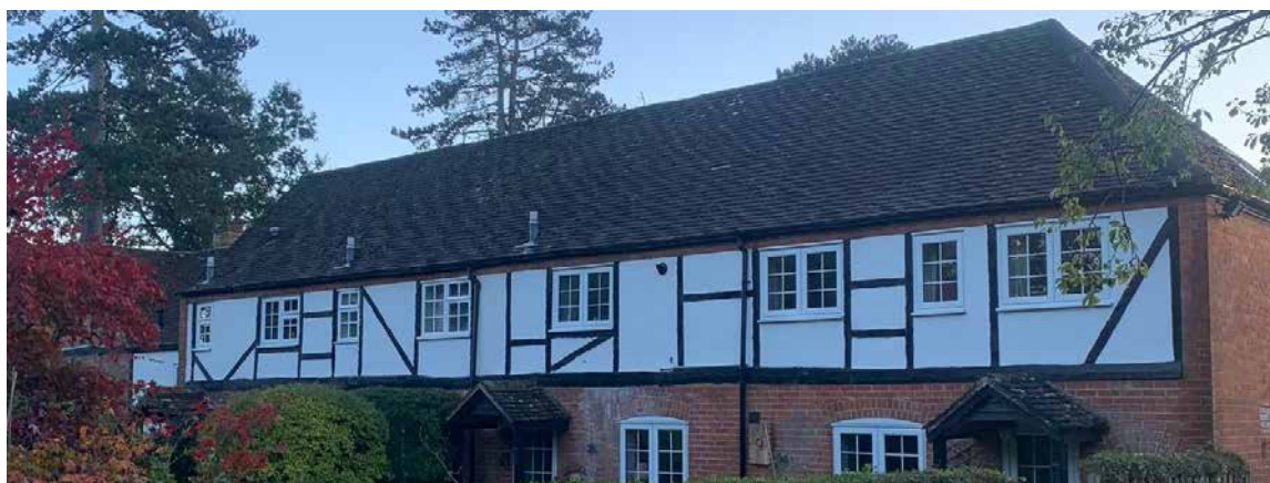
Figure 4 Cottages in Vicarage Lane added in 1st Conservation Area Extension
