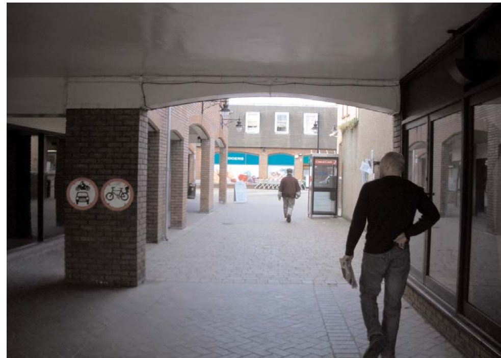
Poor use of greenery or planters leaves the courtyard feeling cold and isolated.
