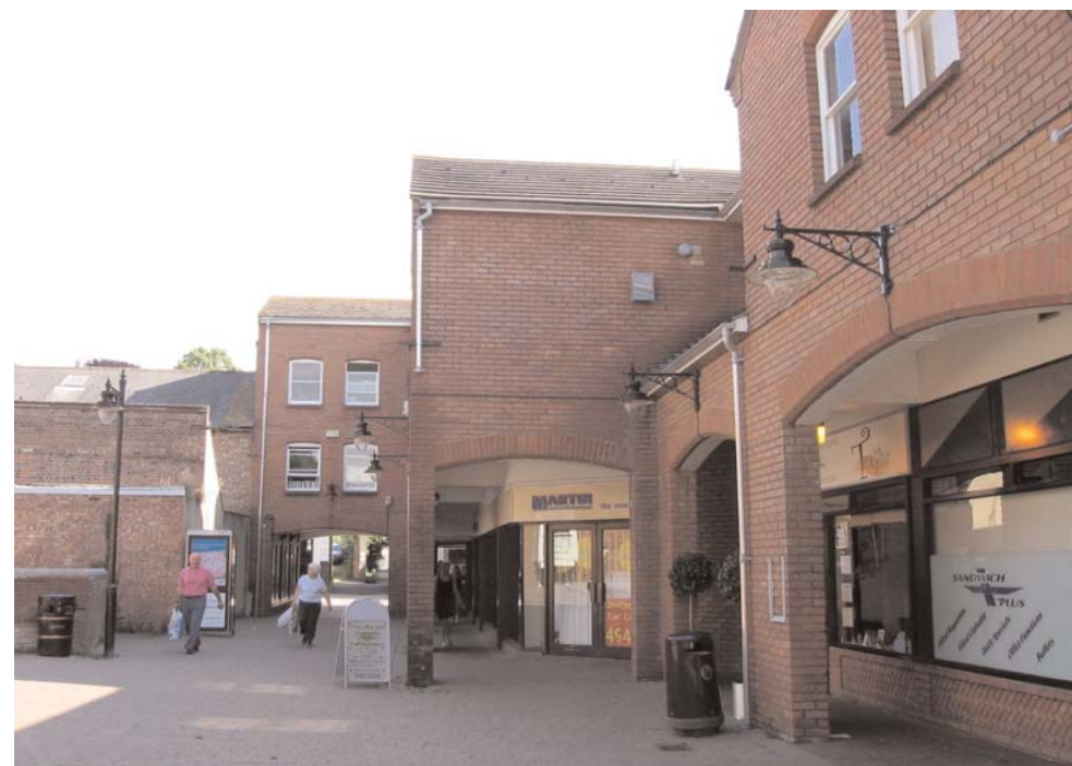
The adaptive re-use of the traditional courtyard morphology provides a new pedestrianised space and provides an active frontage for the shops.
