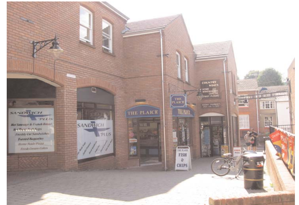
The brickwork is of poor quality and relates little to the late Victorian buildings along the High Street.
