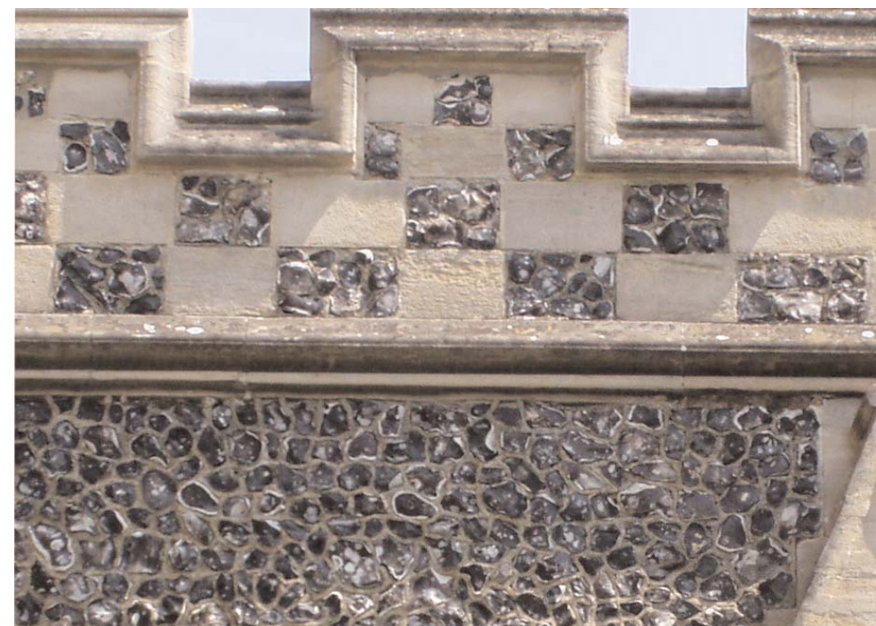
In the absence of good quality sandstone or limestone, flint was used for high status buildings like churches. Limestone was reserved for dressings and mouldings.
