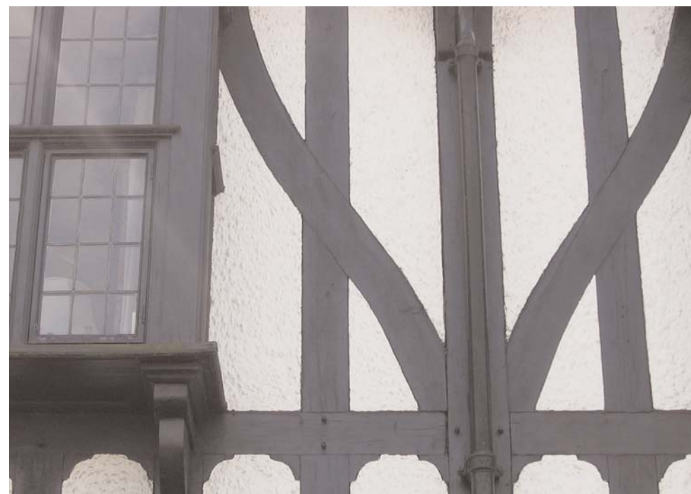
Victorian and Edwardian buildings revived the area's timber-framed tradition, applying plaster and timber for decorative effect.
