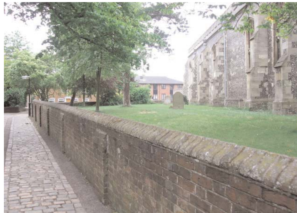
Granite setts are a durable and attractive paving surface but need to be carefully laid to form an even surface. They are traditionally favoured for yards and heavily trafficked areas.
