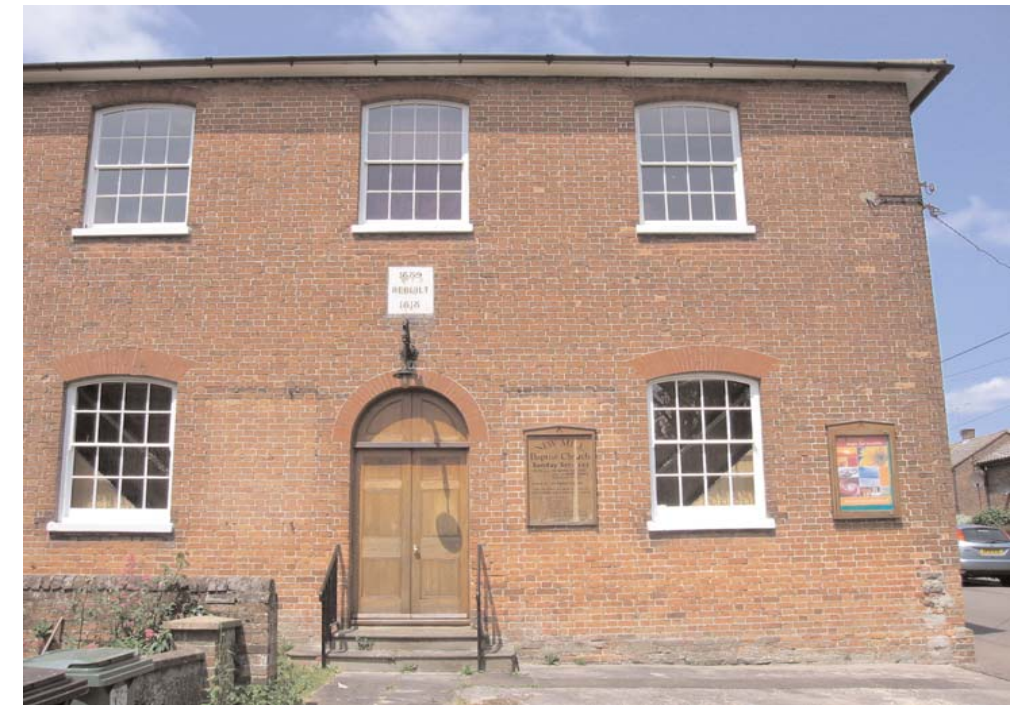
The simple symmetrical facade of the church is enlivened by the use of warm, red brick laid in Flemish bond, with finely cut gauged brickwork over the windows and door.
