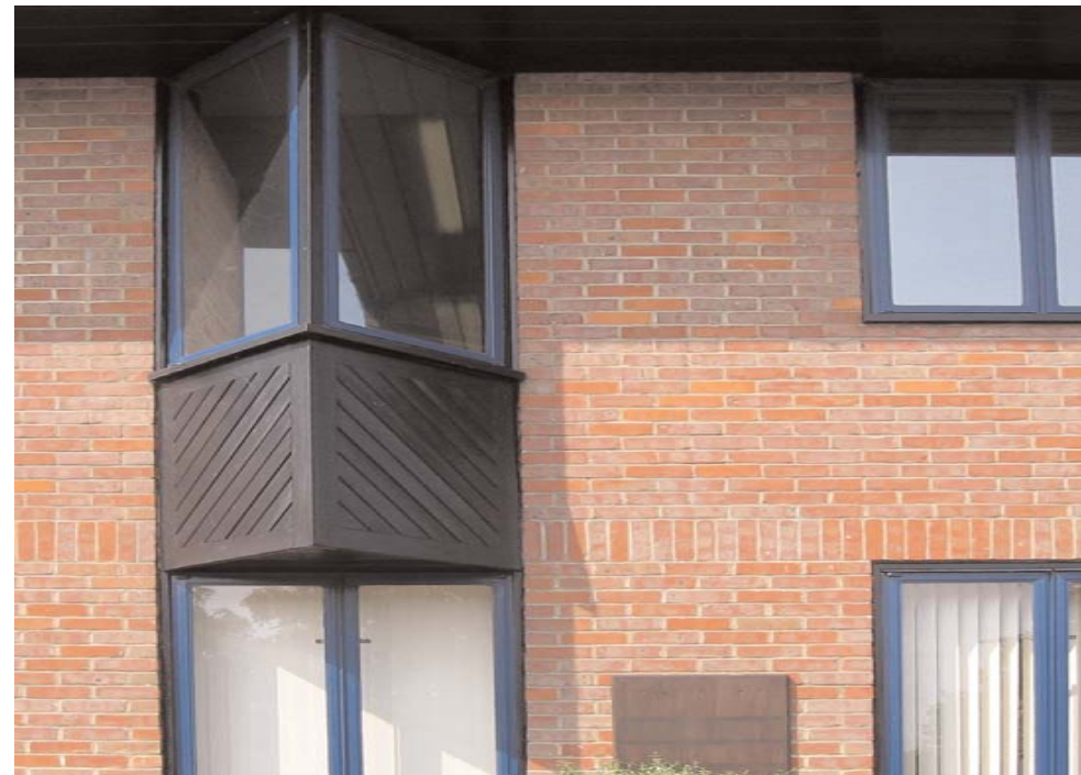
Well detailed contemporary brickwork, using slim red bricks.
