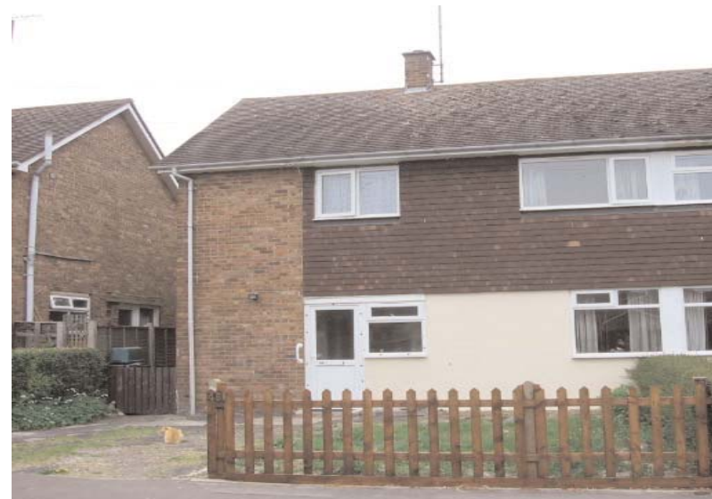
Buff bricks and dark tile hanging were favoured in the 1960s and 70s.
