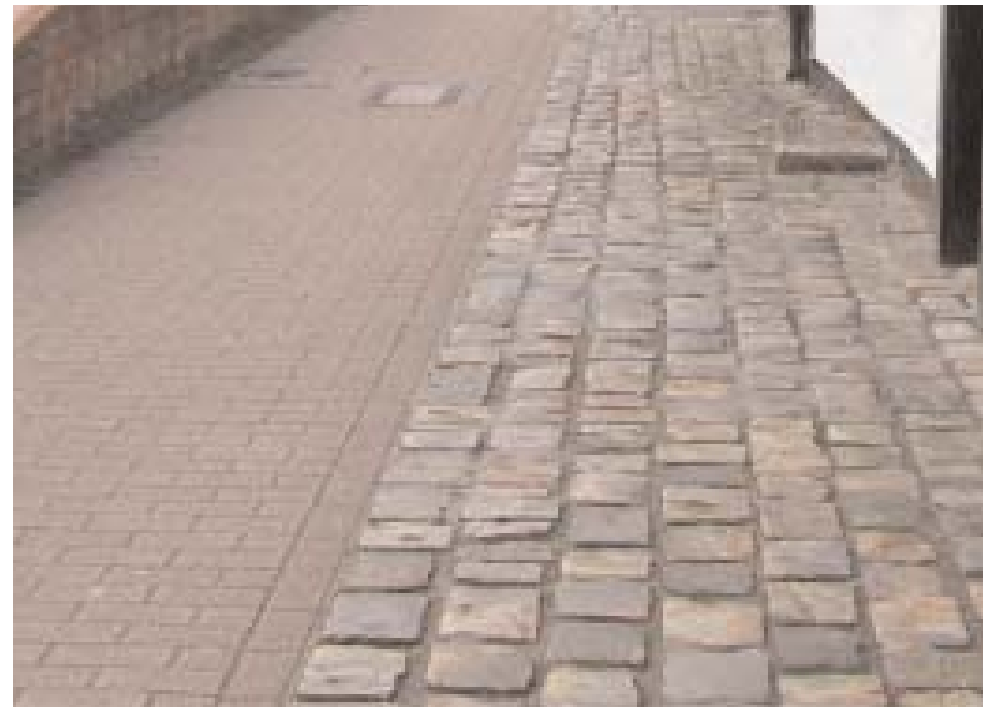
A variety of streetscape elements are used in Tring. The footpath is made up of modern paving bricks adjacent to much older cobblestones.
