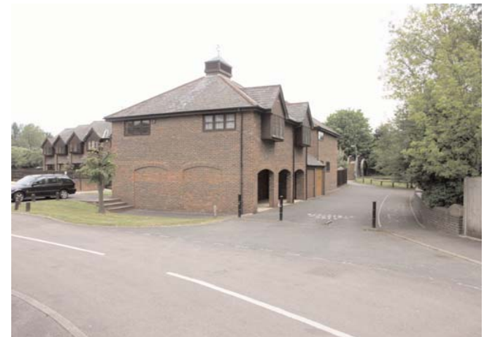
The driveway leading to the left is paved over the River Gade. The use of asphalt leads to increased runoff into the river.
