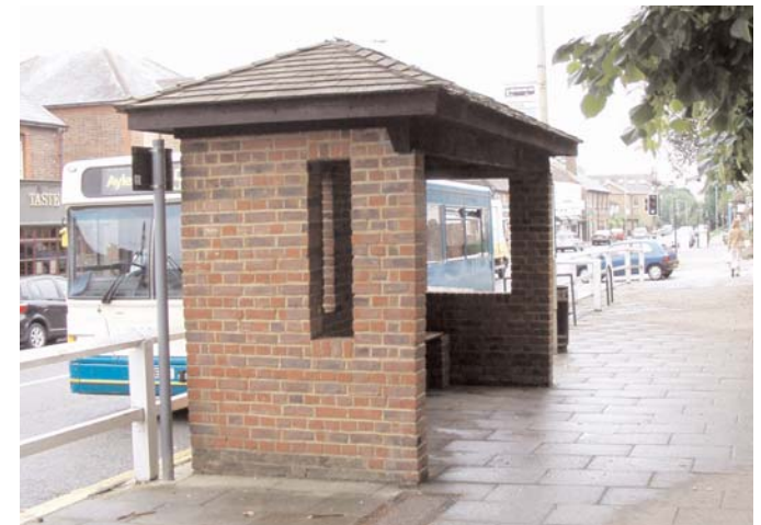
This bus shelter references the village's traditional materials.
