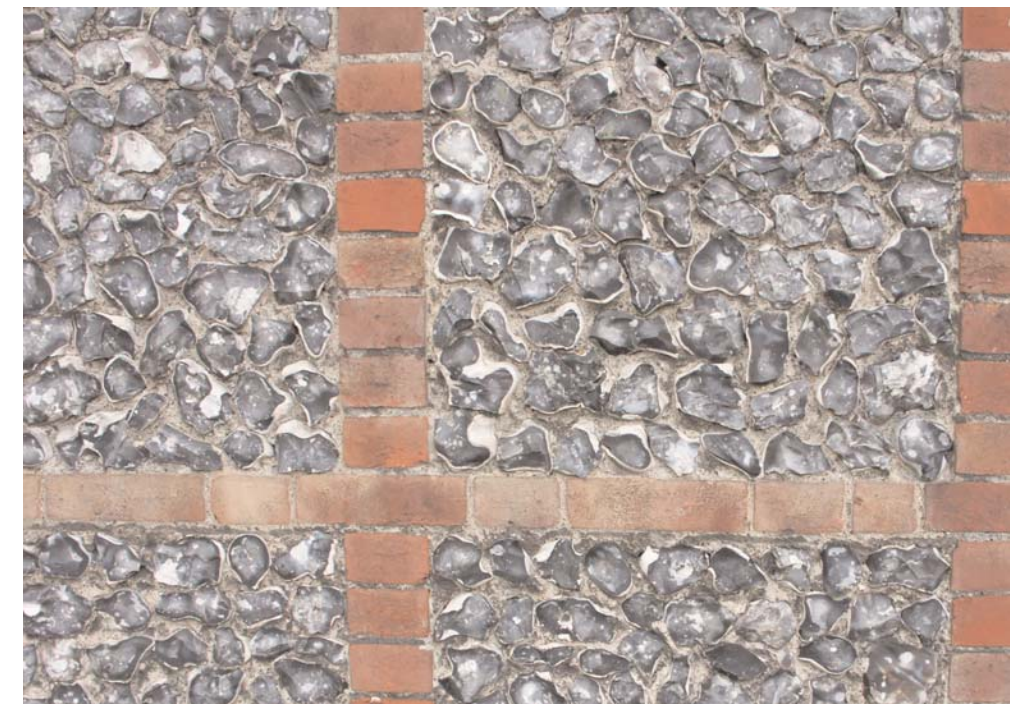
Well laid flintwork can be a visual delight and upholds a local tradition.
