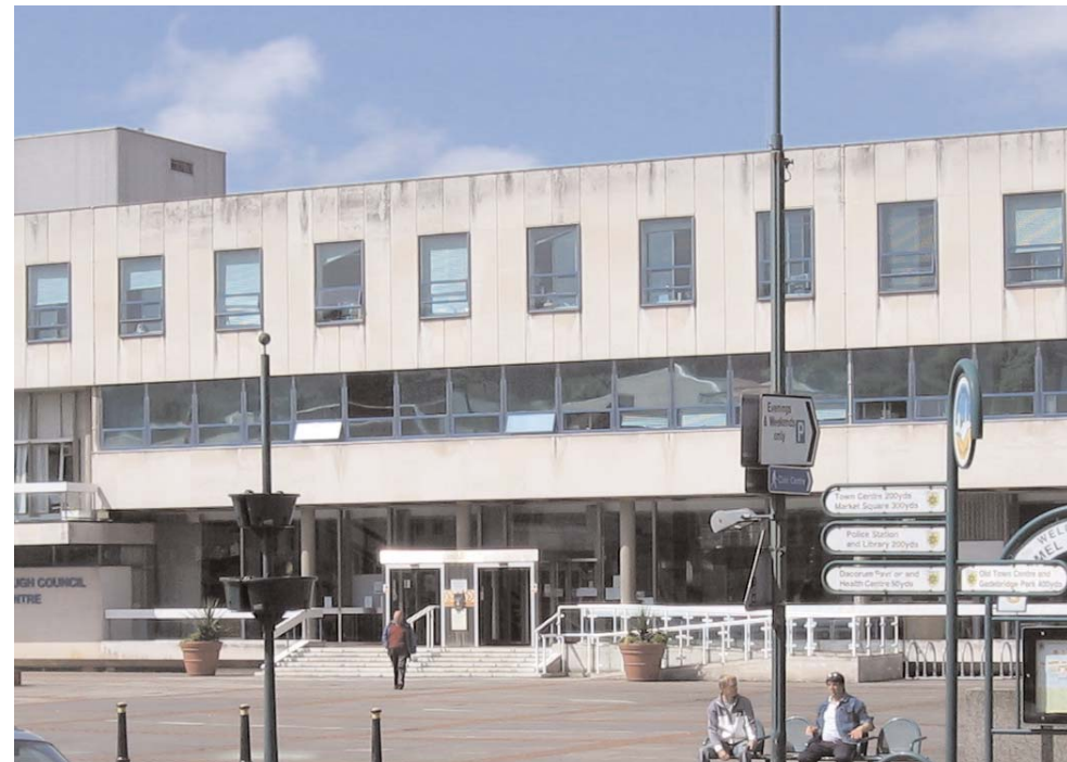
The New Town civic building is of a modernist design with pre-cast concrete cladding (Clifford Culpin Architect 1962-1966)
