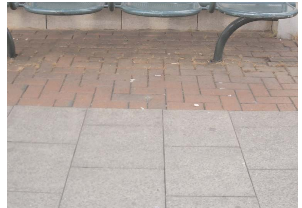
A combination of modern granite slabs and brick in the new town centre.
