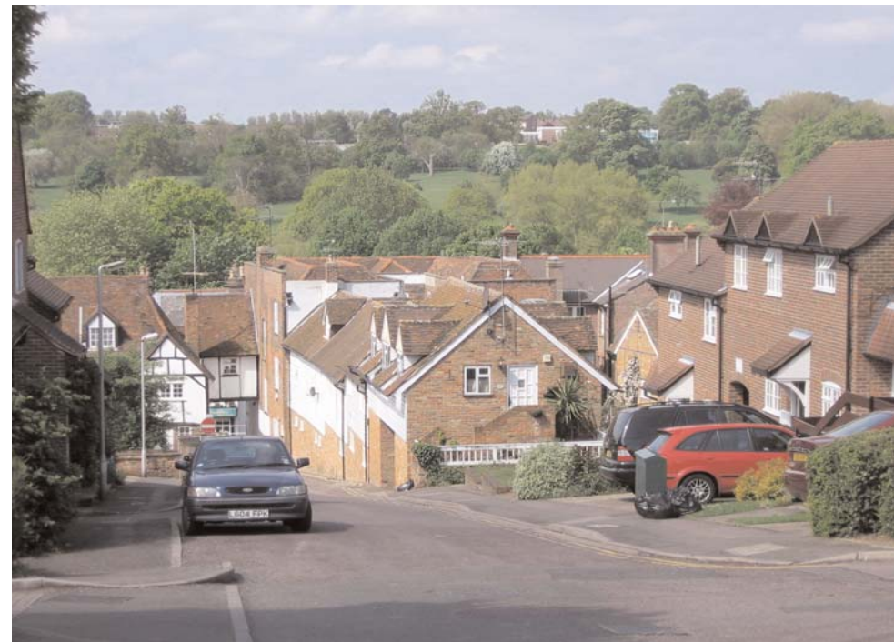
Views across the rooftops towards Gadebridge Park are an important characteristic of the old town.
