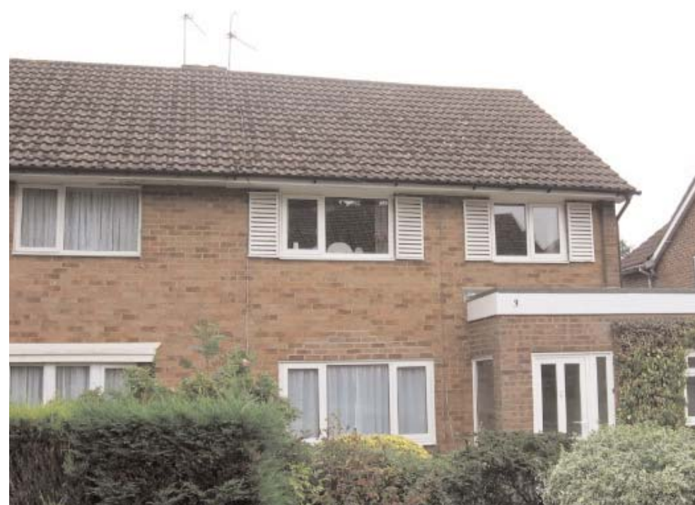
An example of New Town housing with buff brickwork and concrete interlocking roof tiles circa 1970s.
