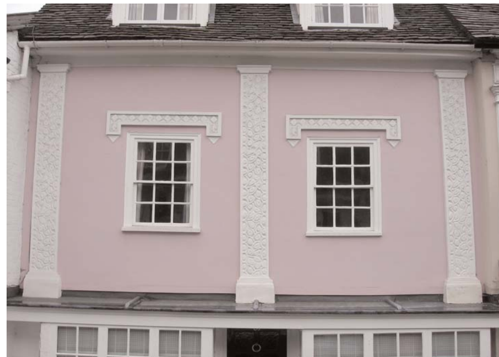
Decorative plasterwork is still to be found in the area, following the East Anglian tradition of pargetting.
