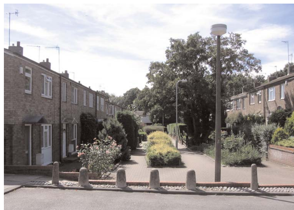
3. Courtyard development with shared front garden private rear garden and off-site parking.
