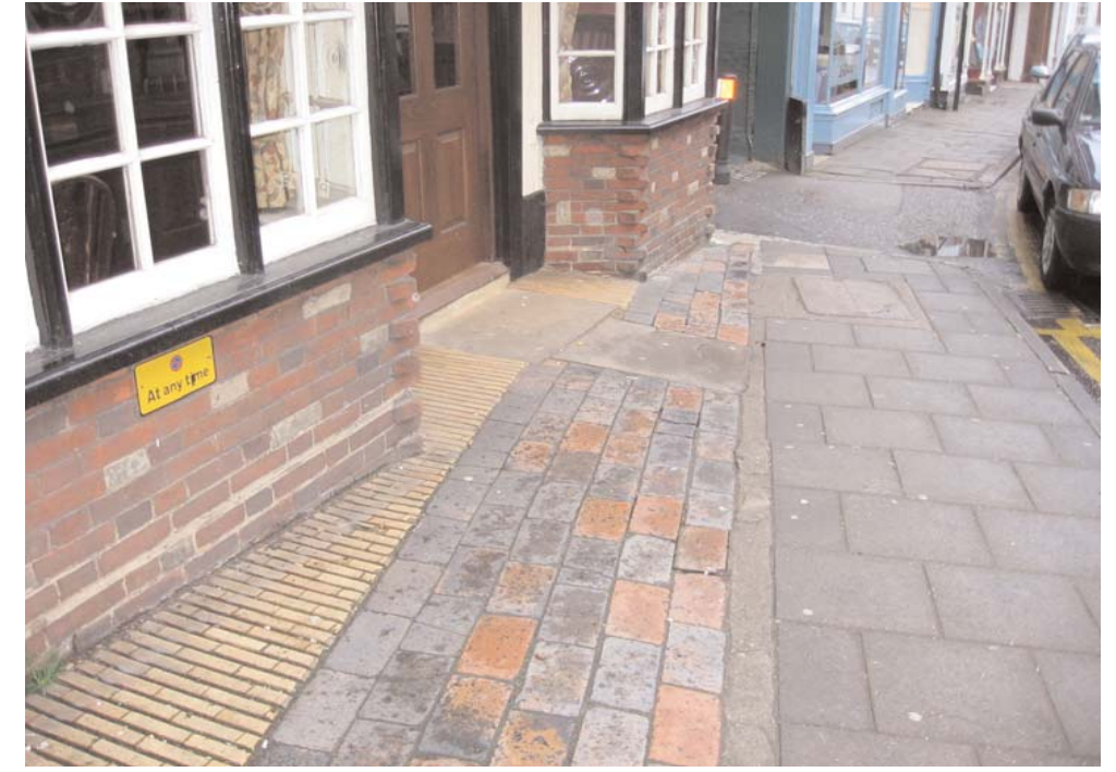
This section of the high street has a combination of clay and concrete pavers.
