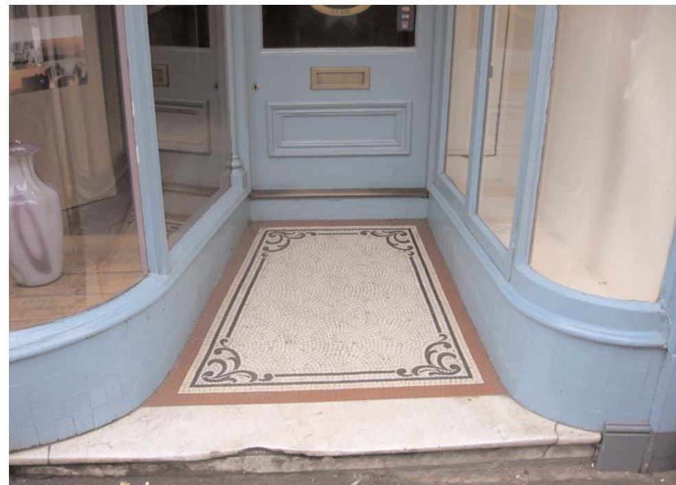
Many shops have Victorian mosaic tiles in the entryway.
