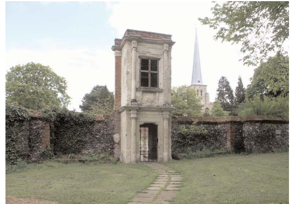
Charter Tower - all that remains of the sixteenth century Bury House. Like the spire of St. Mary's church, it is a cherished local landmark.
