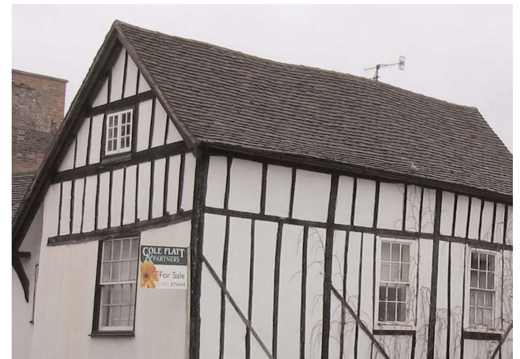
Until the eighteenth century timber framing was the most common building form. The frame was usually concealed behind a coat of lime plaster.
