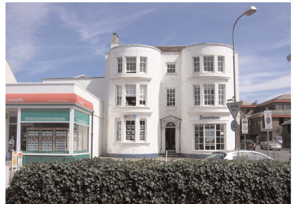
A handsome bow-fronted Regency Villa in Marlowes, compromised by discordant neighbouring development.
