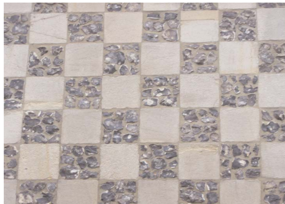
Flint and limestone are sometimes combined to form a picturesque chequerboard pattern.
