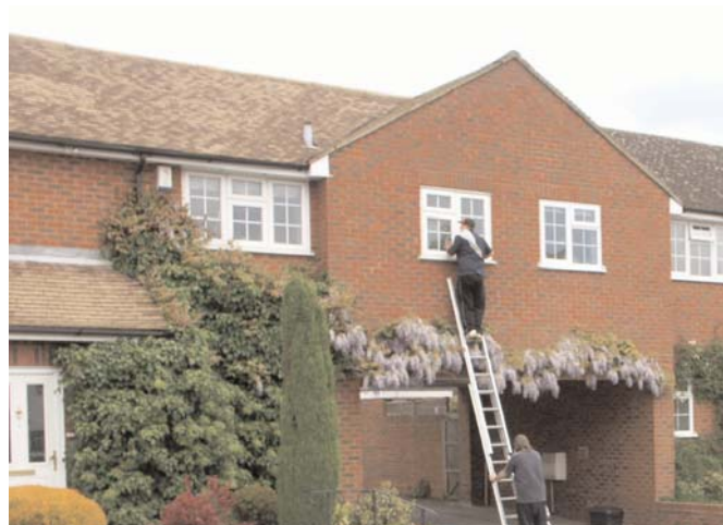
Machine made brick and plastic windows are now commonplace.
