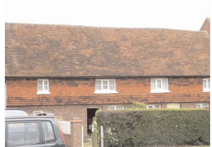
Vertical tile hanging was originally used to protect timber frames but later assumed a largely decorative role.
