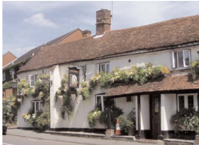
Local brickwork was sometimes limewashed or painted.
