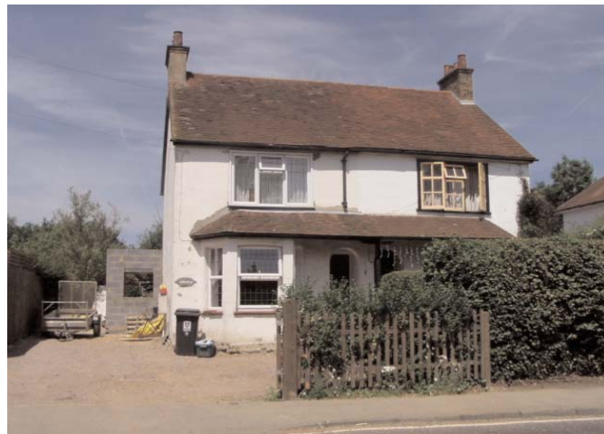
3. Semi-detached with private driveway and front and rear gardens: Green Lane.
