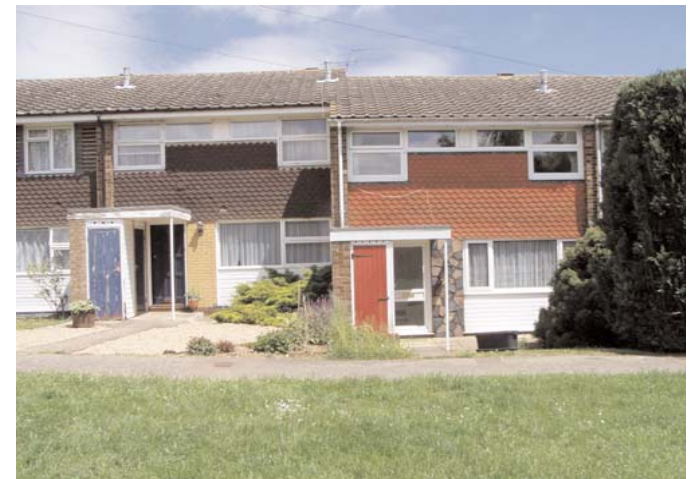
The contemporary use of scalloped tile clashes with surrounding materials.
