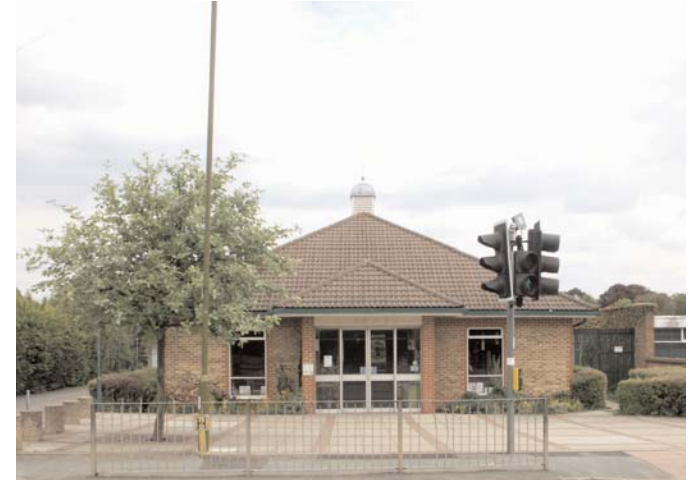
There are few instances of unique paving within Bovingdon. One such area is in front of the library.
