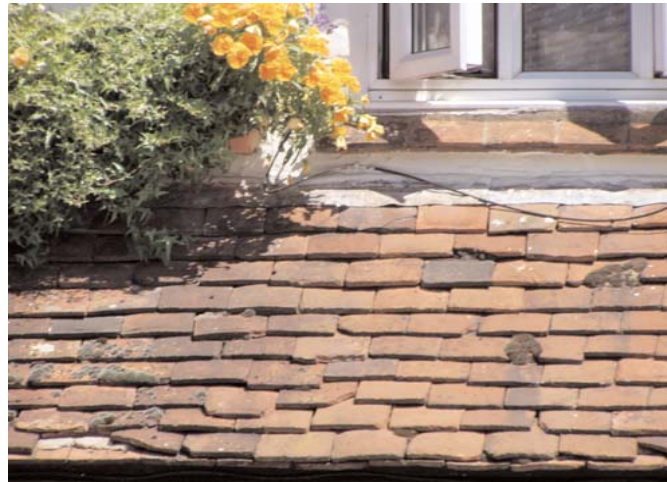
Once thatch ceased to be widely used, hand made plain clay peg tiles were the universal roofing material.
