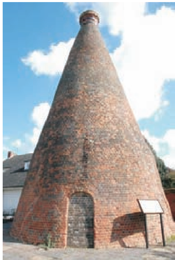
Brick kiln in Nettlebed
