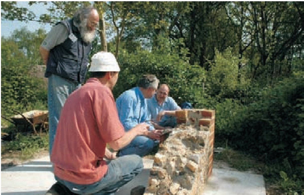
Learning to build a flint wall
